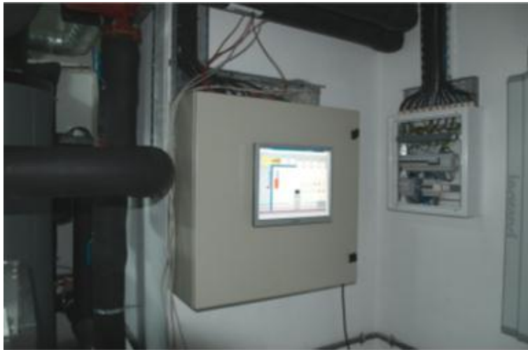
Figure 9: GSHP Measurement and Control System of the GroundMed Coimbra demo site.
