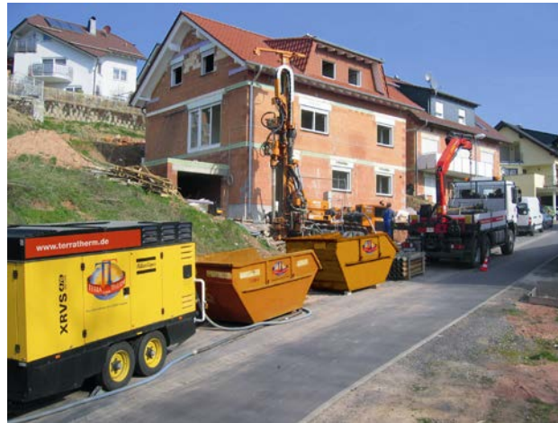
Figure 3. Drilling with down-hole-hammer; to the left the compressor
