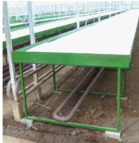
Fig.5. Heating installations positioned below the benches (Vinica, Macedonia)
