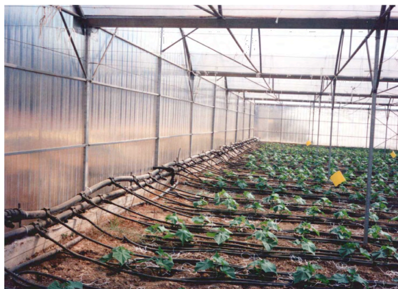
Fig.6. Floor heating installation of corrugated plastic pipes (Xanti, Greece)
