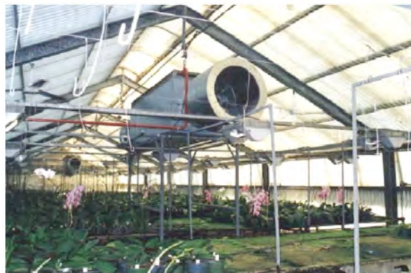
Fig. 7. Air heating system for flowers growing
