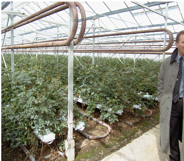
Fig.4. Heating installation of metal pipes positioned above the crop and between the cultivation rows (Vinica, Macedonia)
