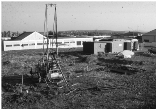
Fig. 2: left: Schwalbach GSHP research station, with light drilling rig, borehole field and buildings for HP and monitoring; photo from January 1988 right: Direct Expansion experiments in Schwalbach GSHP research station in 1989; note ice development on evaporator pipes leading to special BHE
