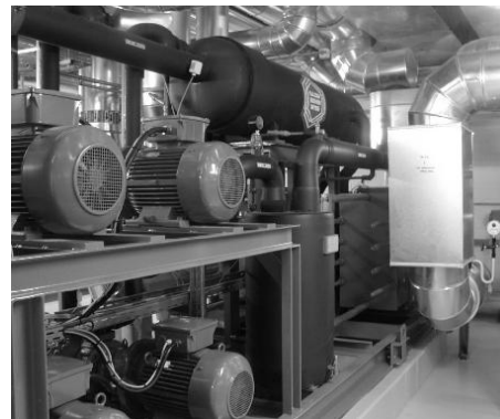
Fig. 15: left: Thermal Response Test equipment on site in Langen right: Heat pump in DFS-headquarters, Langen; to the left four motors driving the compressors. in the background and above evaporator and condensor.
