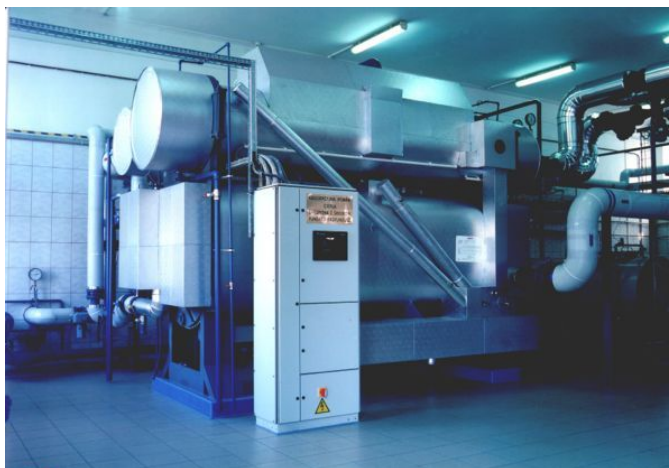
Figure 11. Mszczonow geothermal plant - absorption heat pump (2.7 MW)
