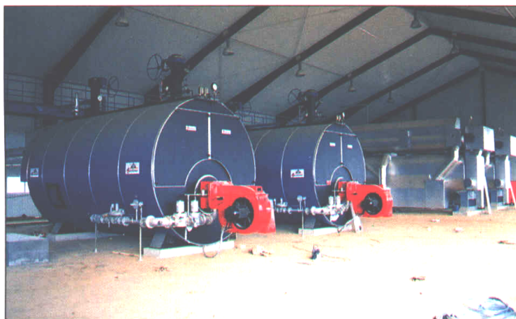
Figure 8. Pyrzyce geothermal plant: natural-gas low-temperature boilers (2 x 10.0 MW) and absorption heat pumps (2 x 8 MW)
