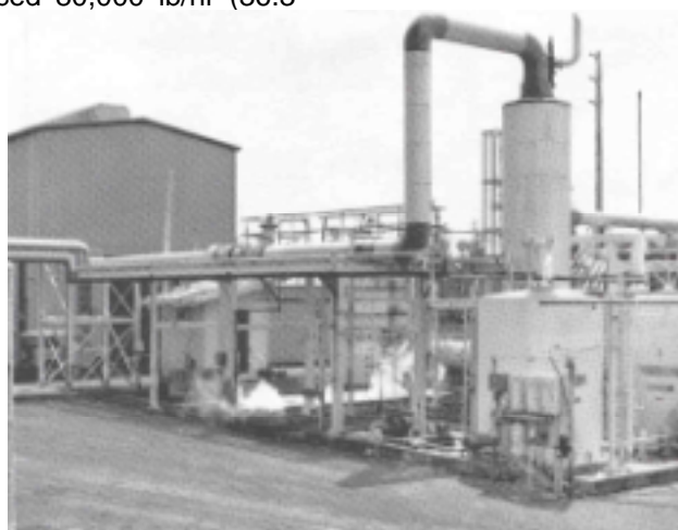
Figure 3. The HGP-A power plant showing the generator building to the left and the steam separator to the right.
