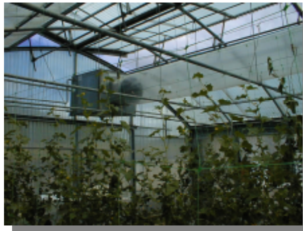
Fig.3. "Fan-jet" geothermal heating system
