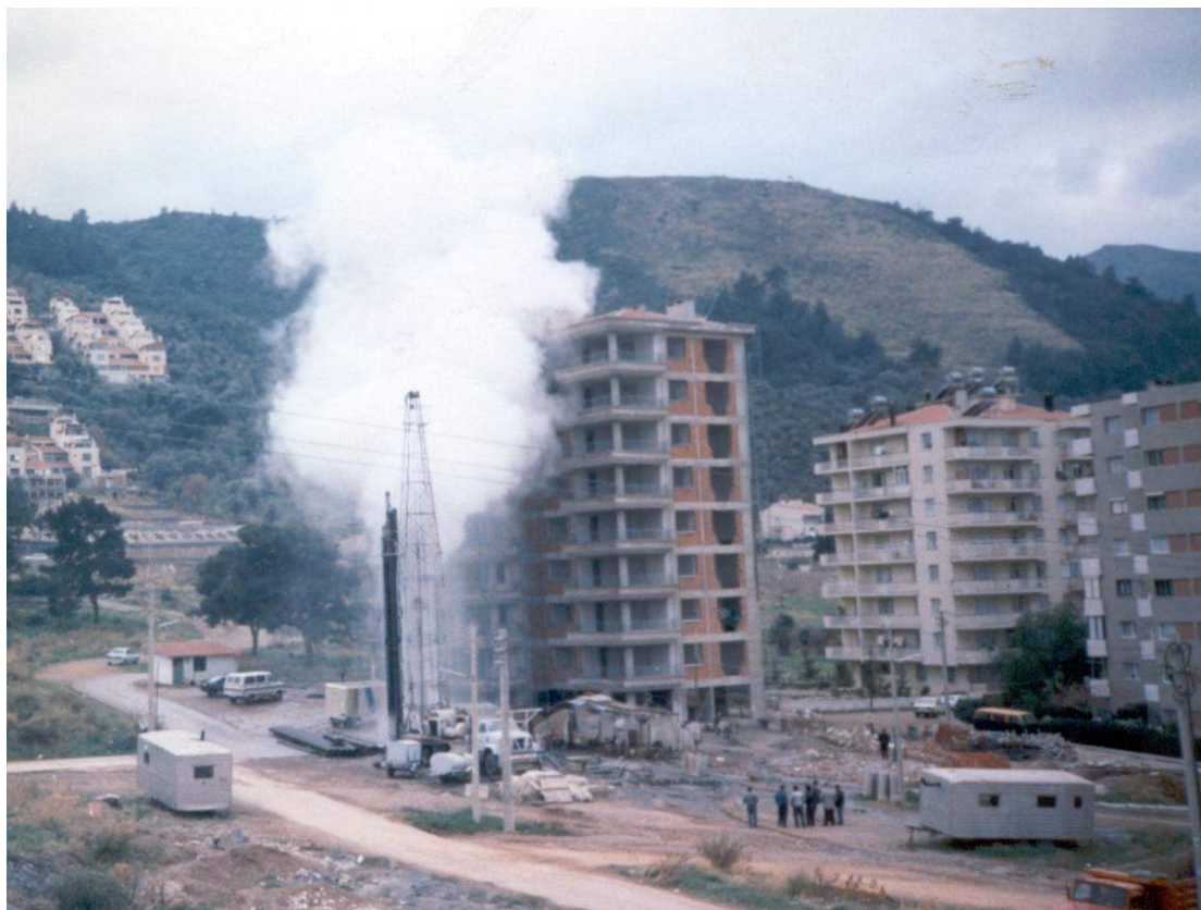
Figure 1: Drilling of BD-3 well in Balcova Geothermal Field in the city
