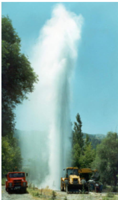
Figure 3: Salihli K-5 Geothermal Production Well, 110 °C, 45 kg/sec
