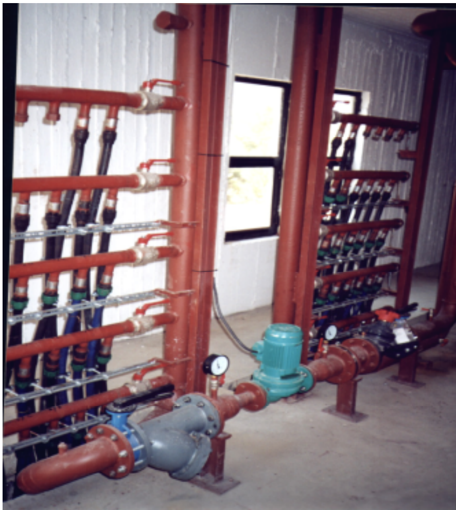
Photo 3: The VEHE system distributors (left) and collectors (right), one of the in-line circulator pumps is also shown.
