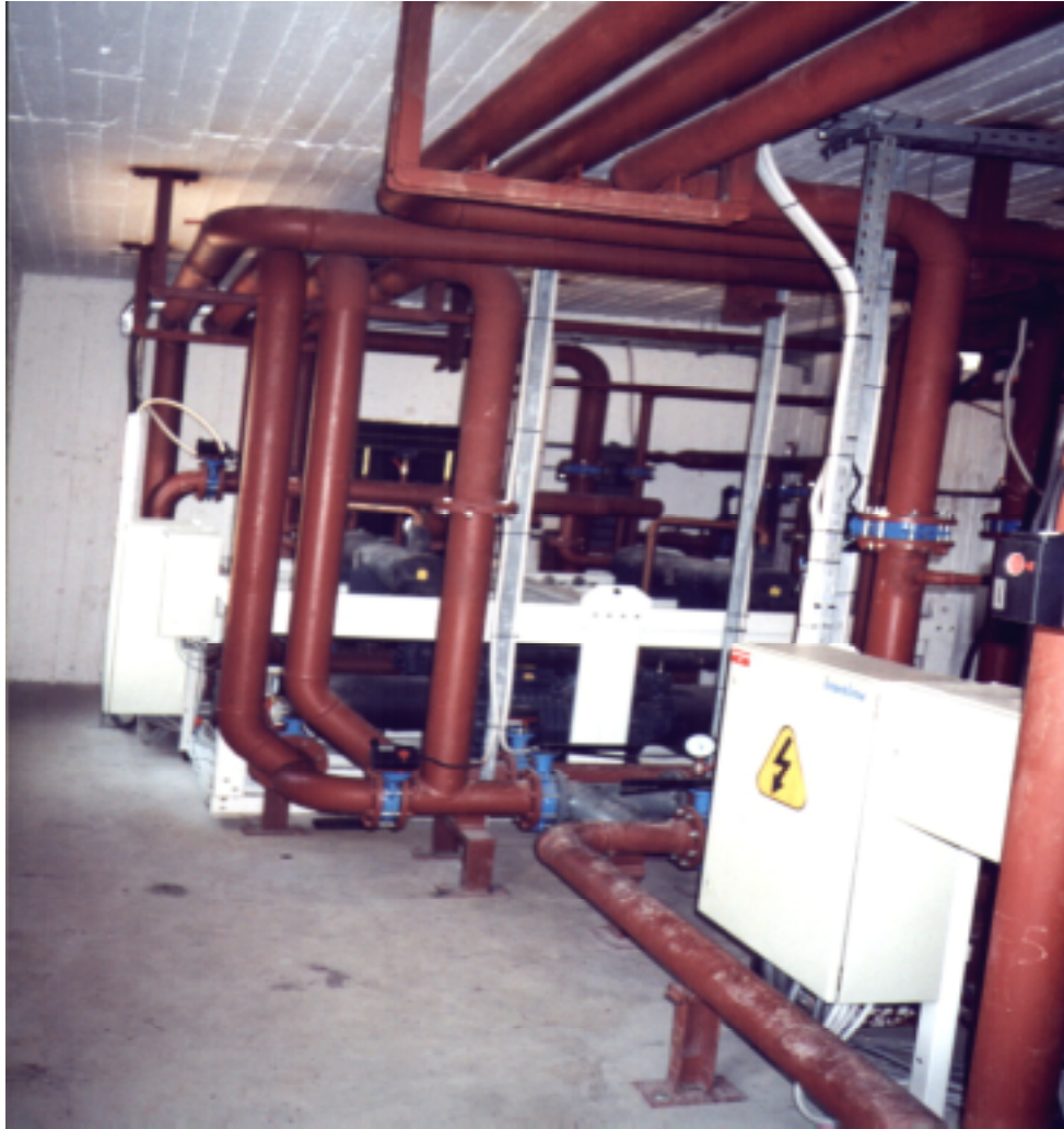
Photo 4: Heat Pump 2, sub-units 1 and 2 (R 22) shown in the distance.
