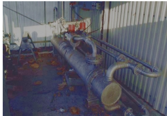
Fig. 14: Main heat exchanger at Wairakei orchid farm.
