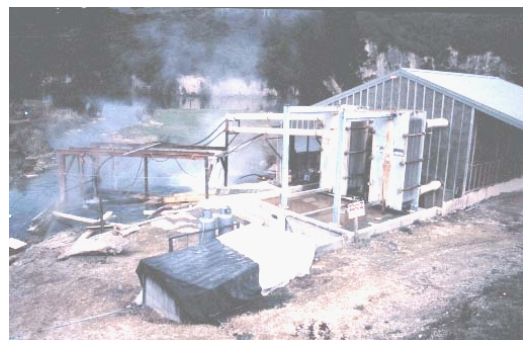
Fig. 8: Hot water intake and plate type heat exchanger at prawn farm, Wairakei.
