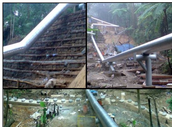
Figure 9. Implementation of the engineering construction Soldier pile as permanent landslide restoration in 2011 - 2012
