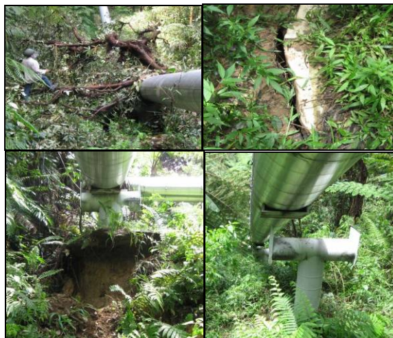
Figure 2. Fallen tree and pipe movement on Awi-14 Awi-2 brine pipeline
