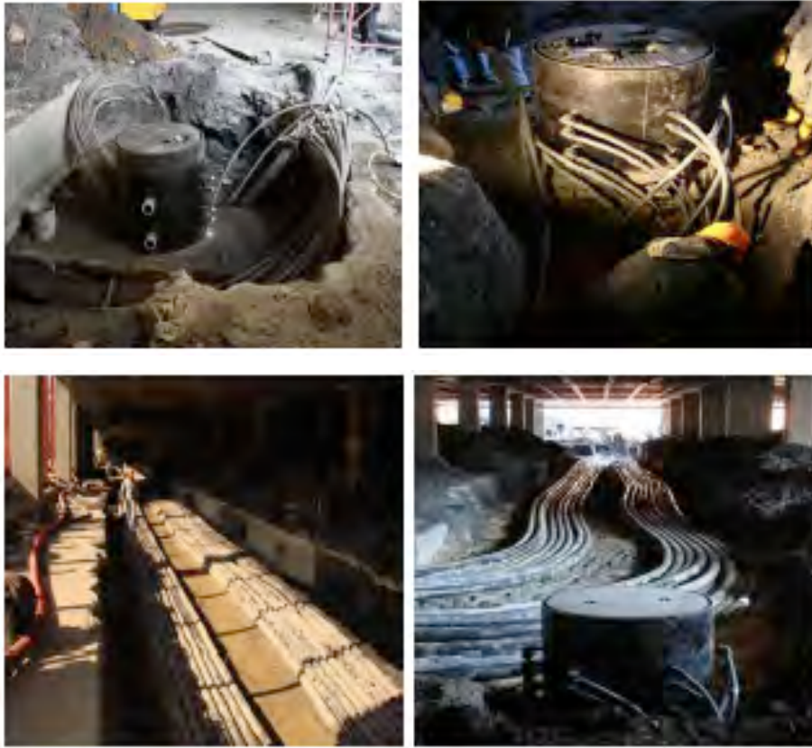
Fig.14-15-16-17 Main piping and collector connections
