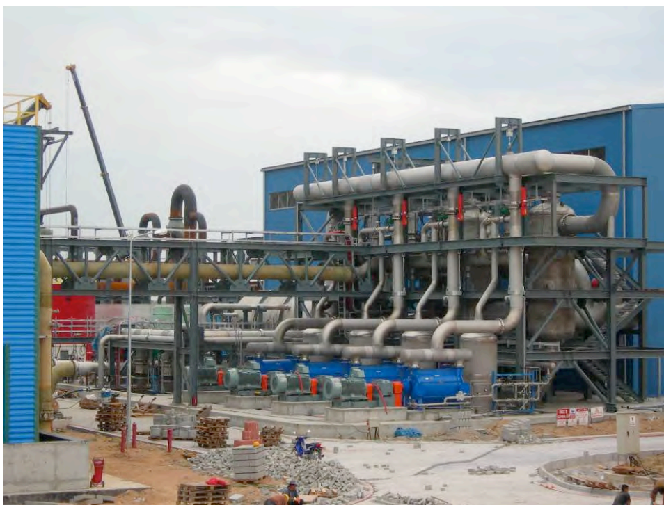
Figure 6. The vacuum pumps (blue components) and ejector trains at Germencik (T. Dunford photo, 2008)
