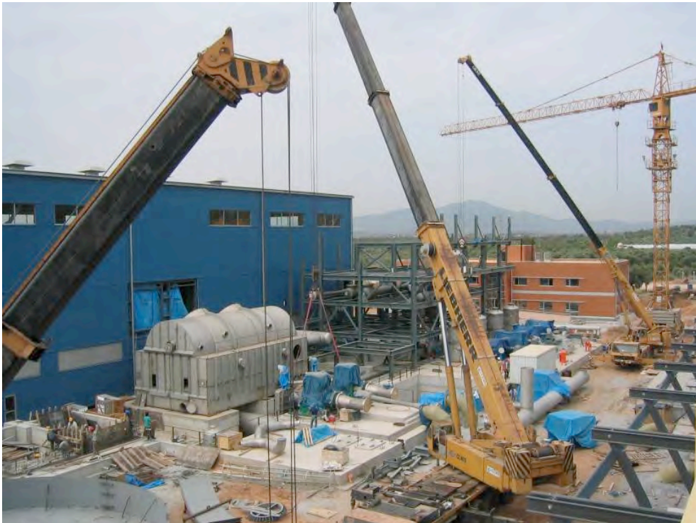
Figure 5: Condenser and Gas Removal System. The condenser is the large drum-shaped vessel just left of center in the photograph.(T. Dunford photo, 2008)
