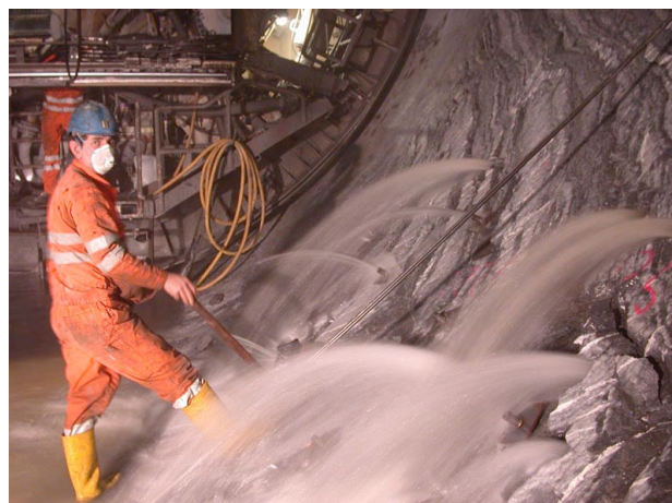
Figure 1 Water inflow in a tunnel (courtesy Matrans)
