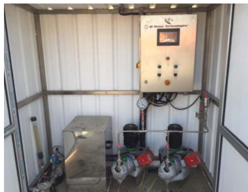
Figure 3: PLC control system, chemical metering pumps and day tank with load cells.
