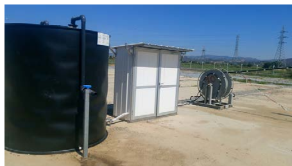
Figure 2: Dilute inhibitor is delivered to a chemical storage tank for wellbore treatment. Protective housing contains inhibitor pumps and control system.
