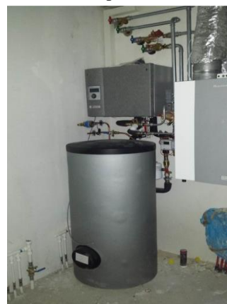
Figure 5. Individual booster heat pump dwelling
