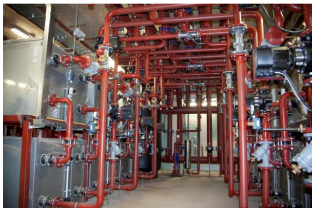
Figure 3. Multiple 2-stage heat pump skids
