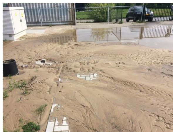
Figure 25. Deformed terrain as result of leakage
