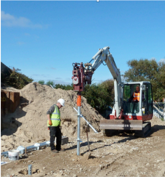
Figure 1: Screw pile installation
