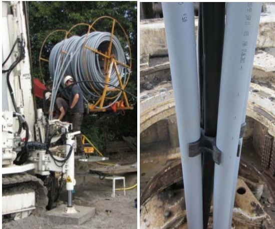
Figure 9: Installation of a BHE with coiler, placed PE-Xa (DN 40 x 3.7 mm)-probe with spacer
