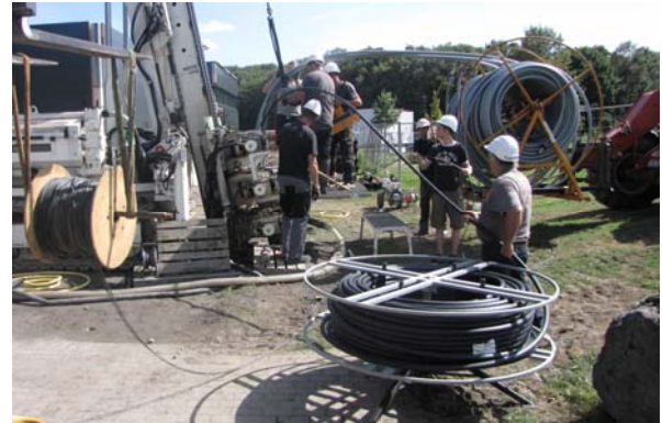
Figure 10: Installation of a BHE with coiler, placed PE-Xa (DN 40 x 3.7 mm)-probe with spacer
