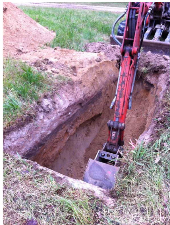
Figure 1: Dredging a test pit at one point of the line the ERT transect was measured on. In Eltersdorf/Erlangen the survey was performed upon sandy soil.
