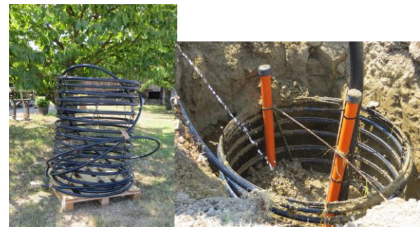
Figure 3: Geothermal basket during realisation phase (a) and buried in the ground, with the pipes allocating the sensors (b).
