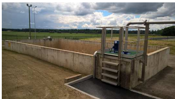
Figure 7: View of rain spool of the Rittershoffen geothermal plant with the transfer pump in case of contamination by geothermal fluid
