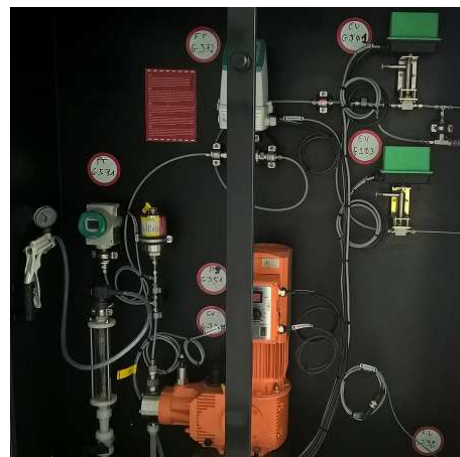
Figure 9: View of the inhibitor injection system on the Rittershoffen power plant
