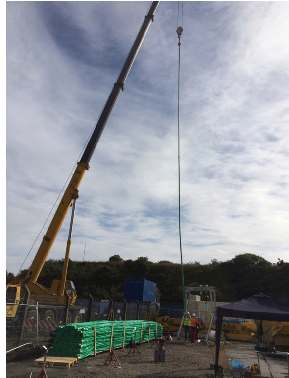
Figure 3 DGSW Pipework being installed at the trial site
