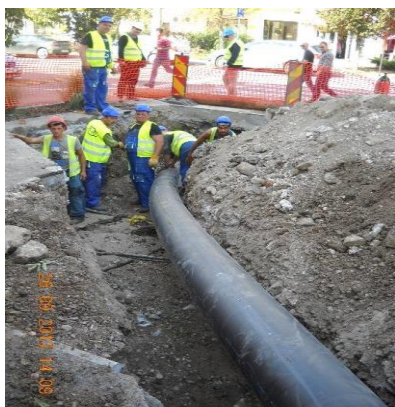
Figure 1. Rehabilitation works of the Otopeni district heating pipeline network [7]
