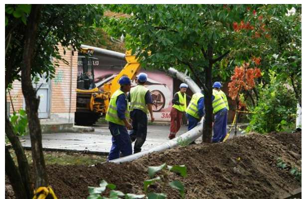
Figure 2: Diameter d225 to d160 installation
