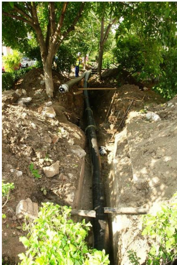
Figure 3: Diameter d225 to d160 installation into existing concrete ducts
