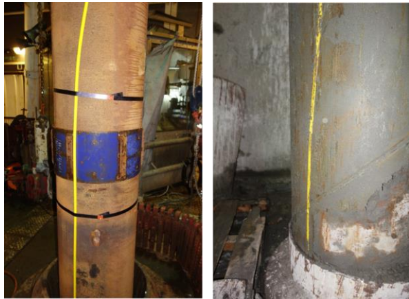
Figure 2: Permanent installation of fibre optic sensor cable behind the anchor casing of well RN-34. Left: during installation, right: cable fully cemented after cementation.
