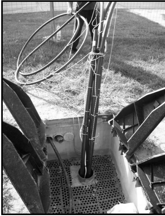
Figure 3: picture of the facility while inserting the heat exchanger.
