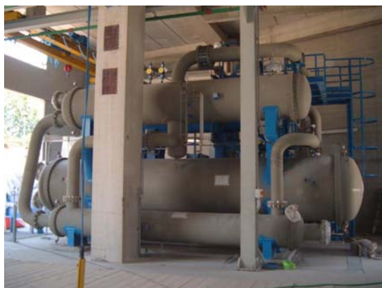
Figure 7: Canaveze heat pump during the installation (2009).
