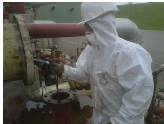
Figure 13: Equipment worn for opening a heat exchanger
