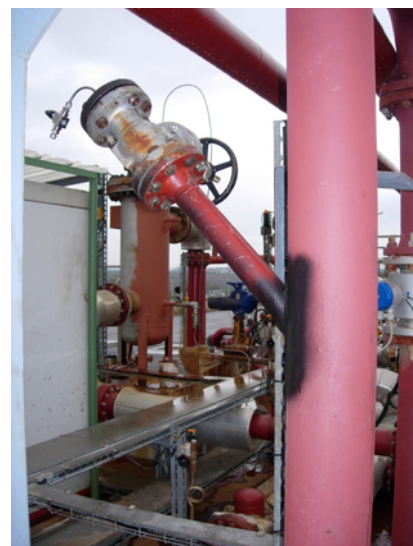
Figure 11: Injection system of the scaling inhibitor located 5 m downstream of the production well GPK-2 (Picture: GEIE).
