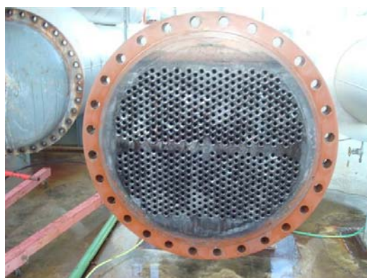
Figure 13: Black scaling observed within the heat exchanger during exploitation.
