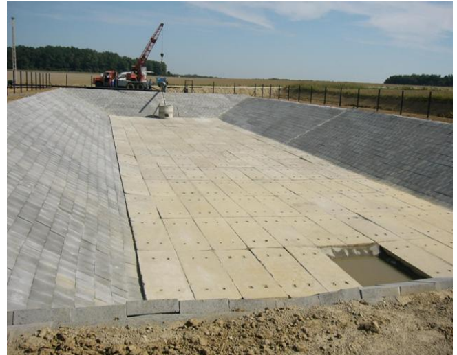
Figure 4: Construction of an environmentally reliable thermal water pit for well testing
