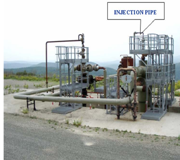
Figure 1: Steam treatment inside well.
