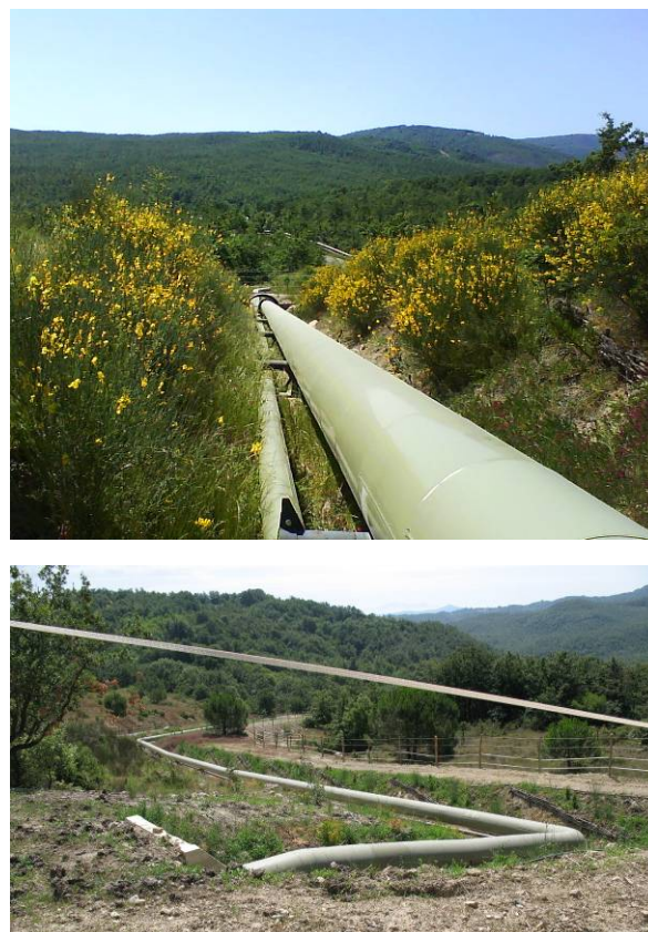
Figure 7: Trenched steam pipelines.
