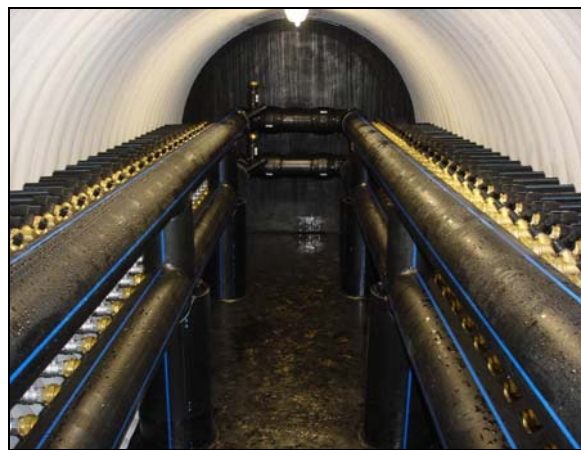
Figure 9: A new type of field manifold, that was first applied at IKEA Helsingborg 2010.
