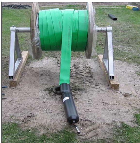
Figure 8: The capsule comes to the site, folded and easy to install with a bottom weight.
