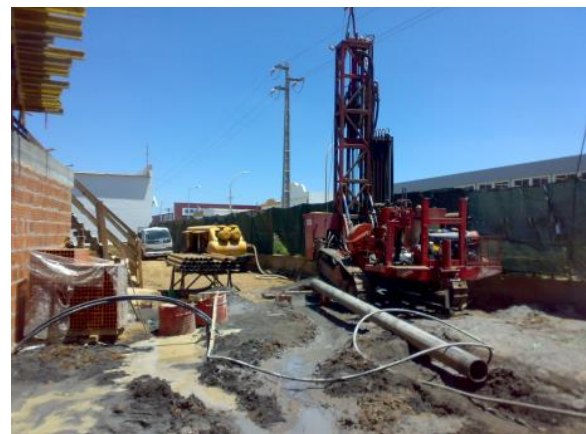
Figure 9: BHE drilling at Sines Business Innovation Centre
