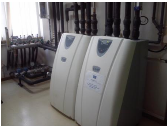
Figure 7: GSHP's installation at EST Setúbal
