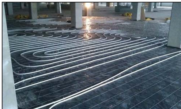
Figure 11. Underfloor heating system
