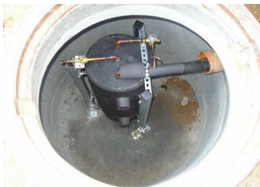
Figure 10: Shaft with installed heat exchanger
