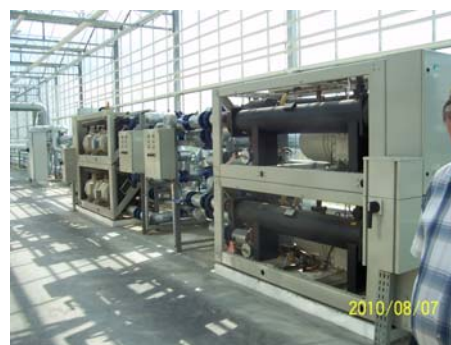
Figure 14: Heat pumps Daikin EWWD 440MBYN at the Greenhouse Complex “Berestyie”.
