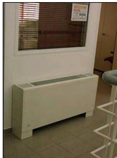
Figure 13: View of a fan-coil in CRES office.
