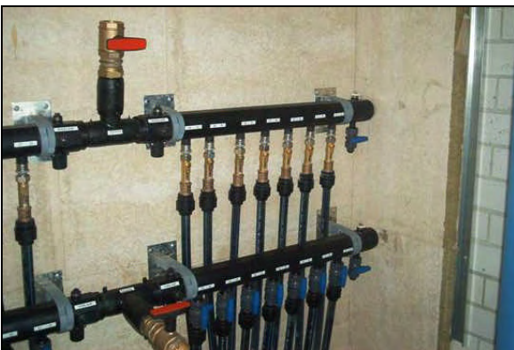
Figure 8: Manifold connecting BHEs to the heat pump(s).
