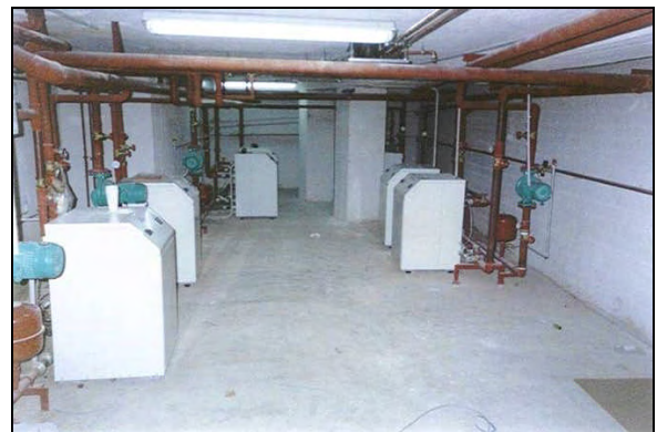
Figure 9: View of water source heat pumps at the Town Hall of Pylaia, Thessaloniki.
