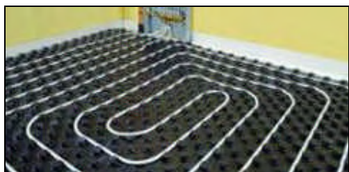
Figure 10: Floor heating system.
