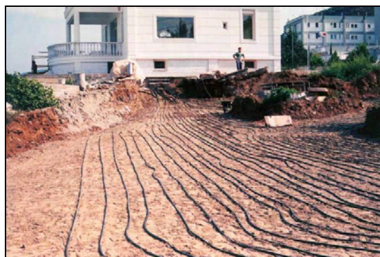
Figure 3: View of a horizontal ground heat exchanger during construction.
