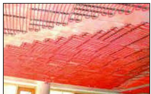
Figure 12: Ceiling cooling system.
