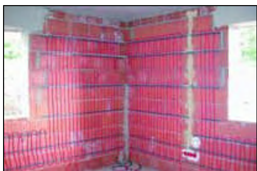
Figure 11: Wall heating/cooling system.
