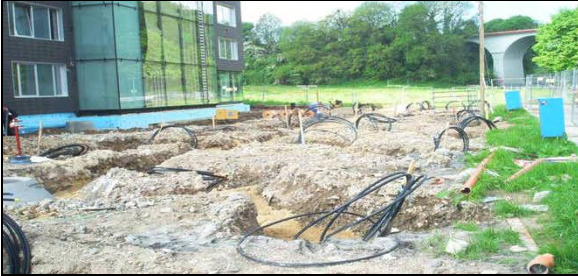
Figure 6: Field of BHEs just after completion (at the German/Belgian border, photo EWS)
