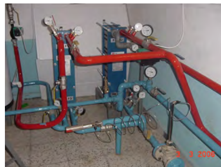
Photo 1: Heat Exchanger System in one of the Buildings in Sarikaya
