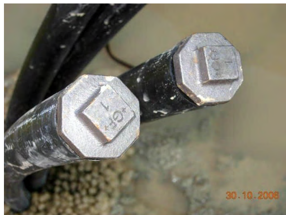
Figure 14: Sealing the BHE's
