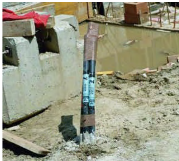
Figure 15: Mark and protect the BHE against damages.
