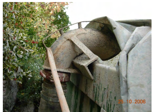
Figure 12: drain off the cuttings into a hutch using a safe transportation hose
