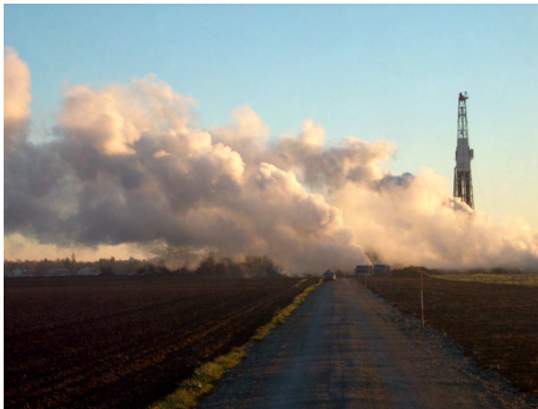
Figure 1: Successful pump test of the second drilling in Unterhaching. The temperature of the water found in more than 3 km depth is about 130°C.
