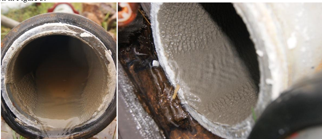
Figure 5. Inspected alvenius lines after increased GSX dosing to 8ppm
