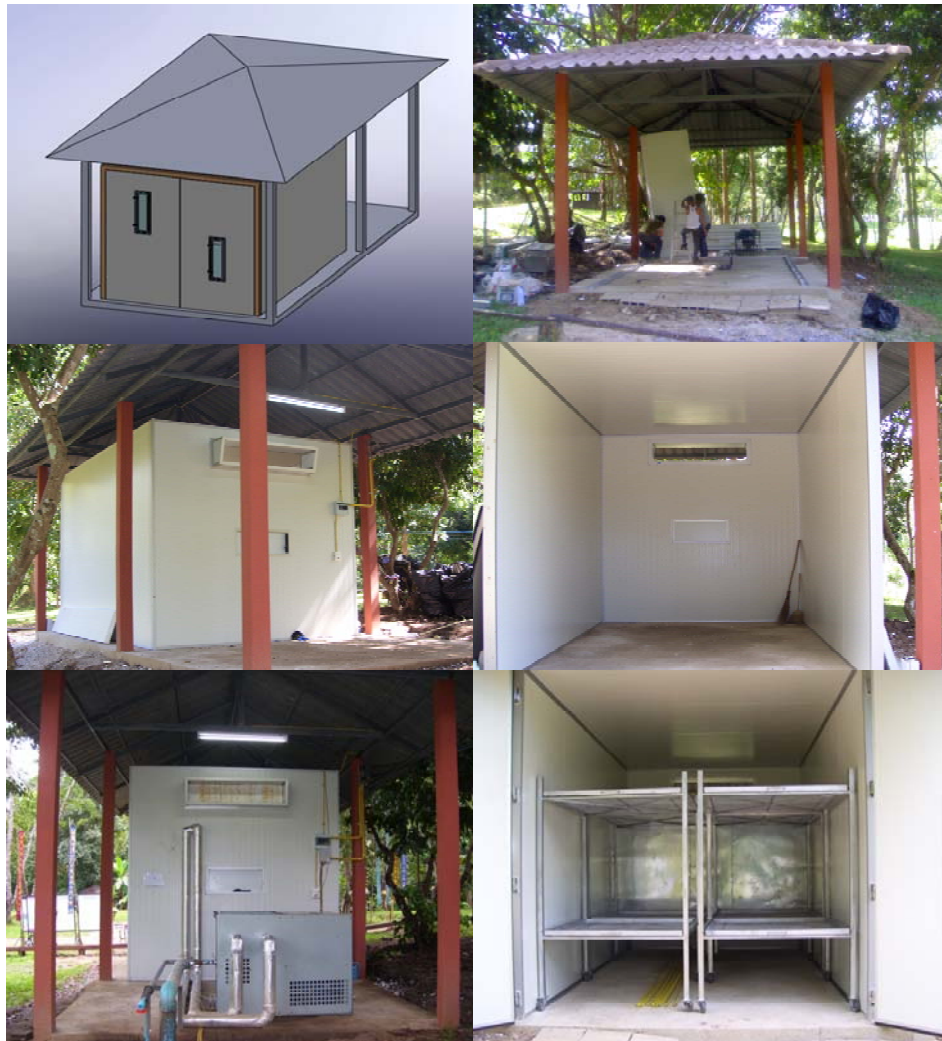
Fig. 7 Drying room with the heat pump system.
