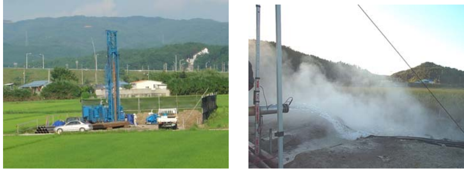
Figure 7. Drilling rig for test well BH-2 (left) and geothermal water developed from BH-2.
