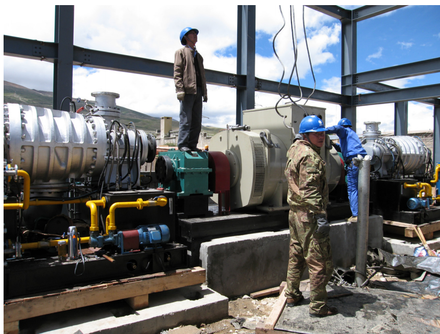
Fig. 1 1,000 kWe screw-expansion engine installed in Yangbajain geothermal power station in Sep. 2008
