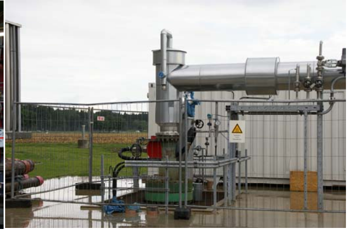
Fig. 2 A 3.4 km deep production well in the Unterhaching geothermal power plant, Germany, 8 August 2008 (Photo by Muraoka).
