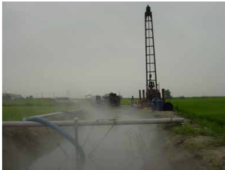
Figure 4. Drill rig and overflowing waters from 1,280 deep well at Seokmo-Do.
