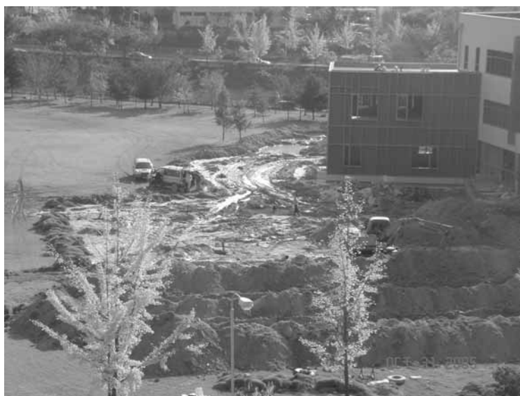
Figure 5. Trenches and double U-tubes for borehole heat exchanger for Earthquake Research Center building at KIGAM.
