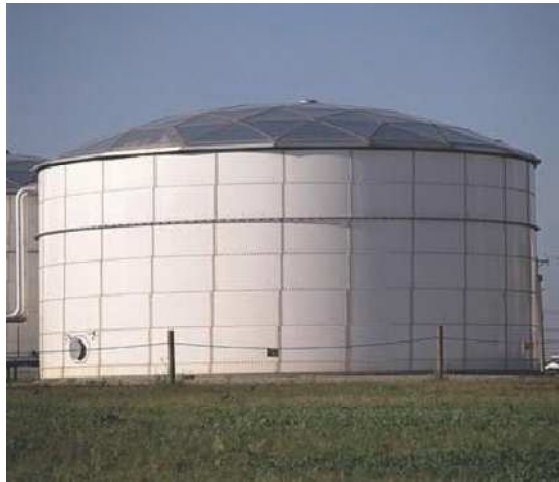
Figure 2: A typical steel panels bolted tank
