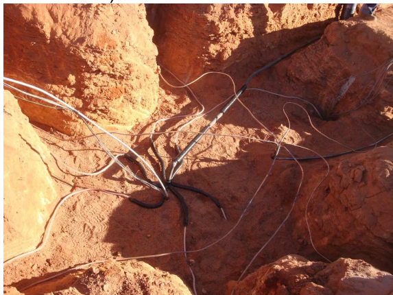
Figure 1: Loops, liquid & vapour manifold and trenches.
